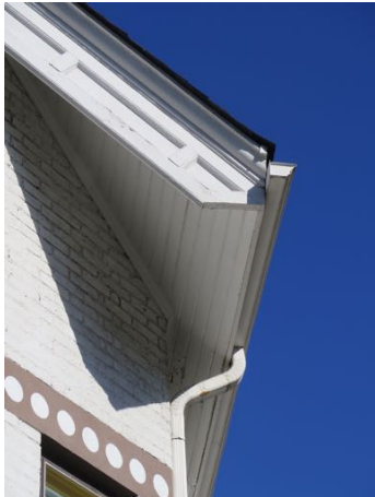
Fig 28, West elevation bargeboard and soffit
