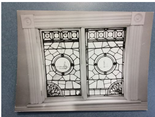
Fig 26, 1970s photograph of window (North elevation)
