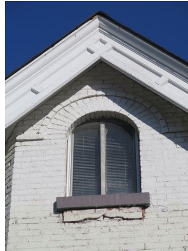
Fig 25, Arched window with brick detailing (replacement window)
