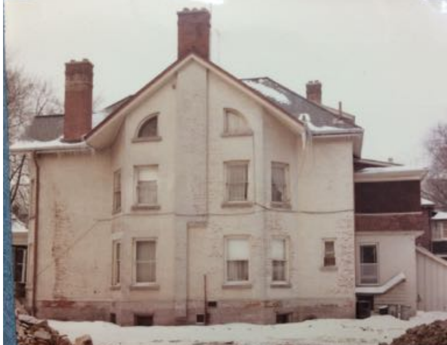
Figure 15, 1963 Photograph of 11 Madison Avenue after the demolition of 9 Madison Ave
