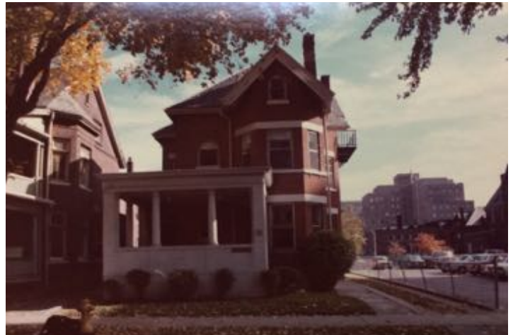
Figure 17, 1970 Photograph of 11 Madison Avenue
