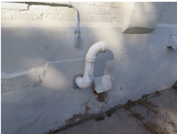
Fig. 22, Above grade foundation wall, parged (South elevation)
