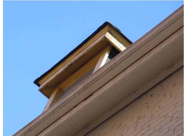
Fig 29, North elevation wood dormer and soffits
