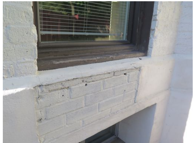
Fig 23, Visible brick at water table line, at modified window (South elevation)
