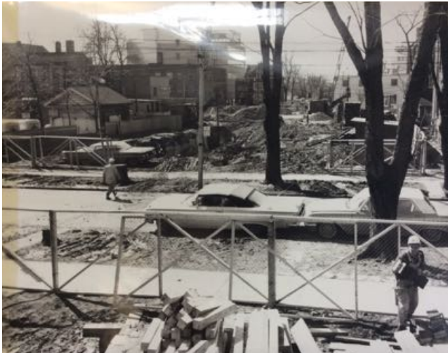
Figure 12, 1964 Photograph showing Subway construction
