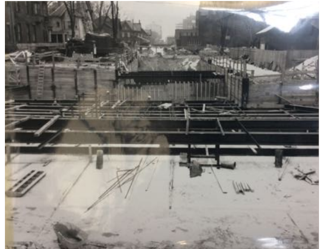
Figure 13, 1964 Photograph showing Subway construction
