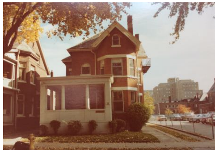
Figure 19, 1974 Photograph of 11 Madison Avenue
