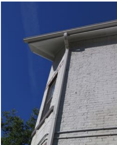
Fig 30, Rainwater leader and eaves trough on southwest corner
