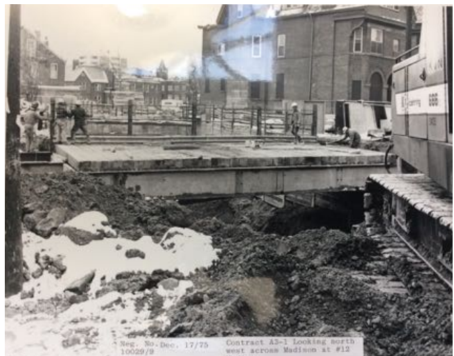
Figure 13, 1975 Photograph showing Subway construction
