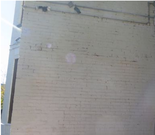
Fig. 20, Masonry wall, (East Elevation)
