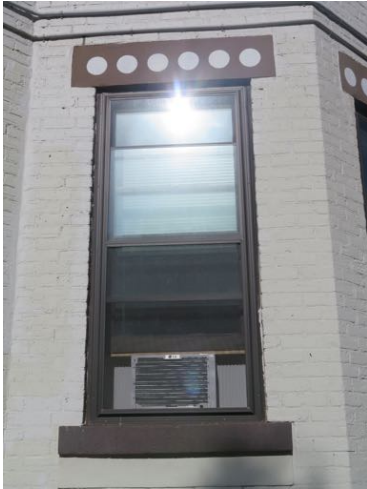
Fig. 24, Exterior of typical window with aluminum storm
