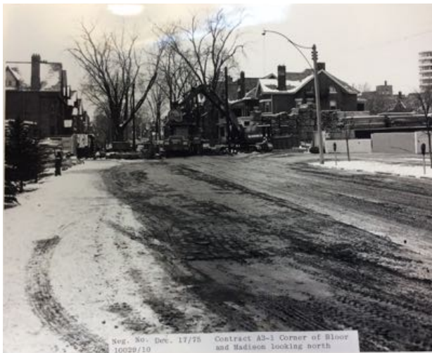
Figure 14, 1975 Photograph showing Subway construction
